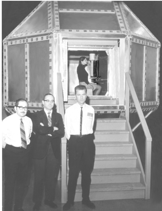
Figure 1. (L to R) Ed Edelsack, myself, and Jim Zimmerman at the MIT shielded room, in Dec. 1969. The first low-noise MCG had been recorded here a day earlier, using Jim's SQUID. "Laurie", at Ed's request, poses as a subject in front of the long-tail glass dewar, which contains the SQUID.
